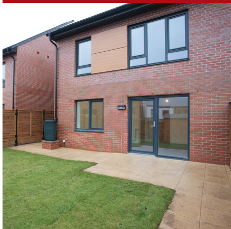
Contour Homes and Keepmoat Ltd eco-trial. House built to Code Level 6 of Code for Sustainable Homes.
